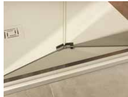
Close up of Opening
